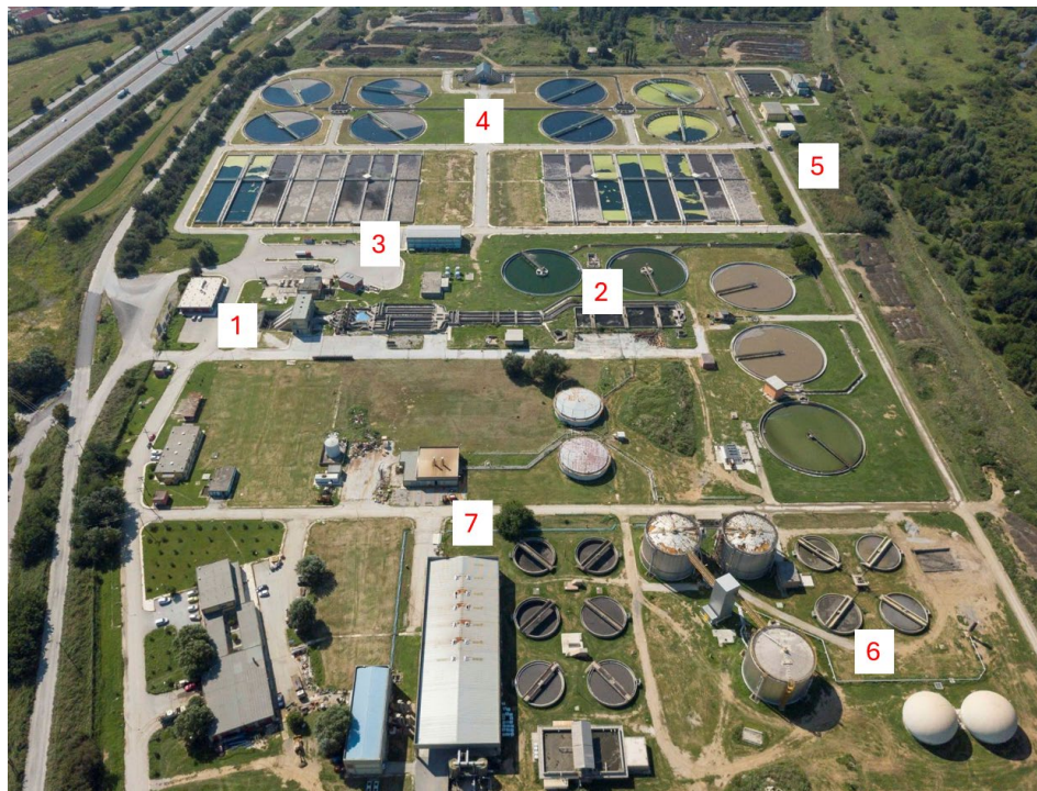
Figure 11: The Wastewater treatment plant of Thessaloniki
